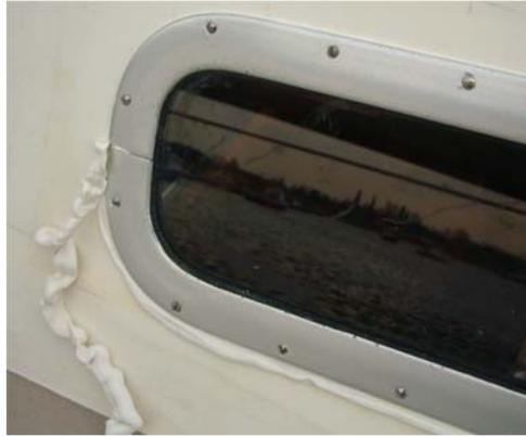
Figure 14: Trimming Surplus Window Sealant
