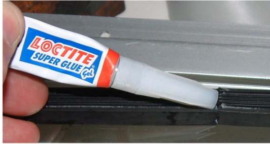
Figure 7: Bonding Rubber Seal
